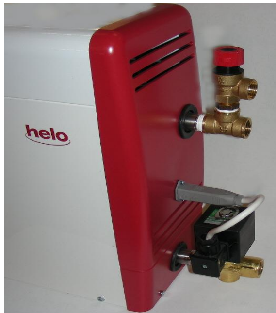
Image. Installation of the safety valve and the automatic drain valve
